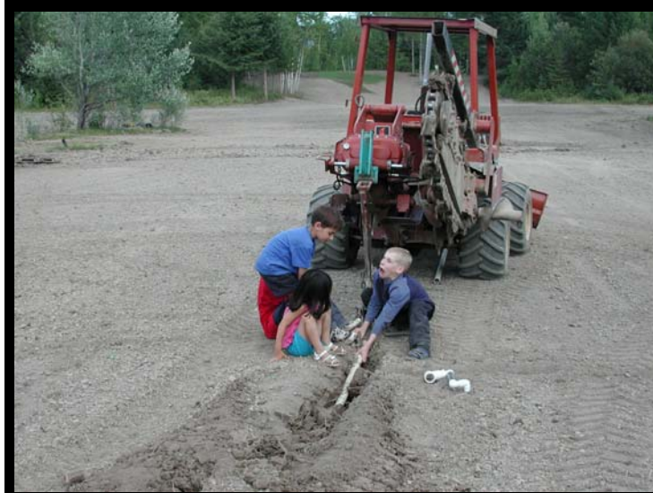
Pulling Irrigation lines for Fairway #2
